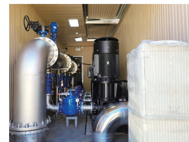
The outdoor one-stop water pump that can be operated through the Internet — Huang Jiaying
