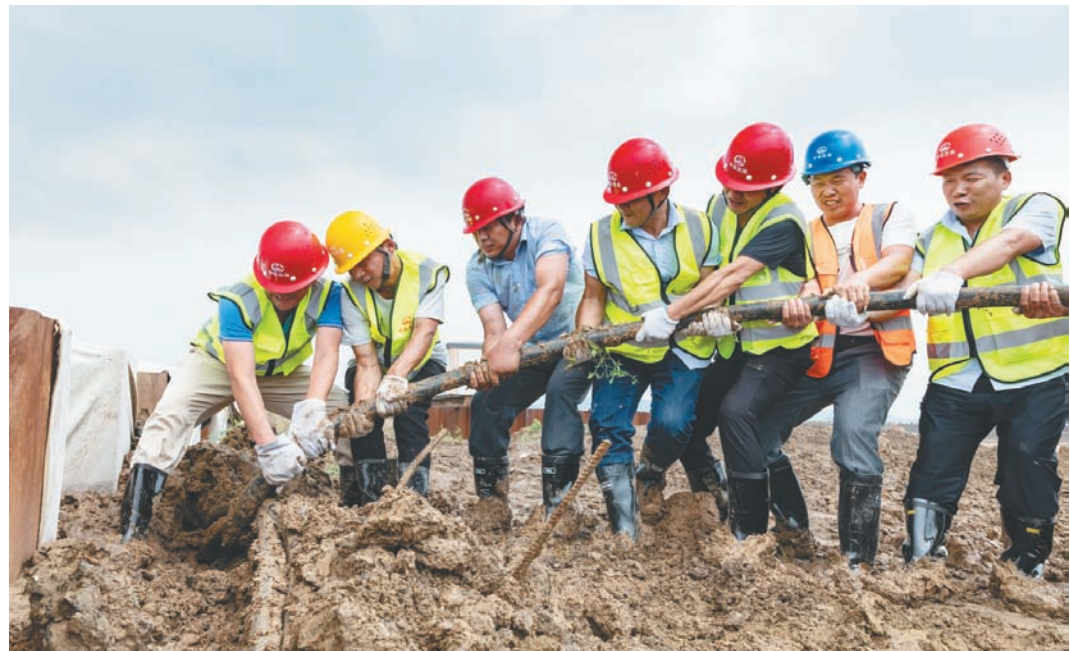
“党员突击队”在铺设高压电缆
