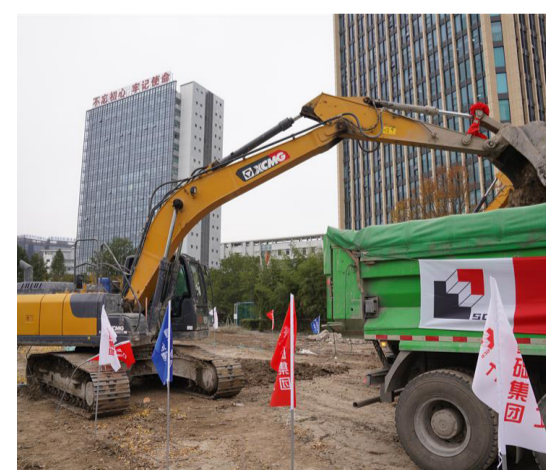
Construction starts at the Dongjing Metro Station.
